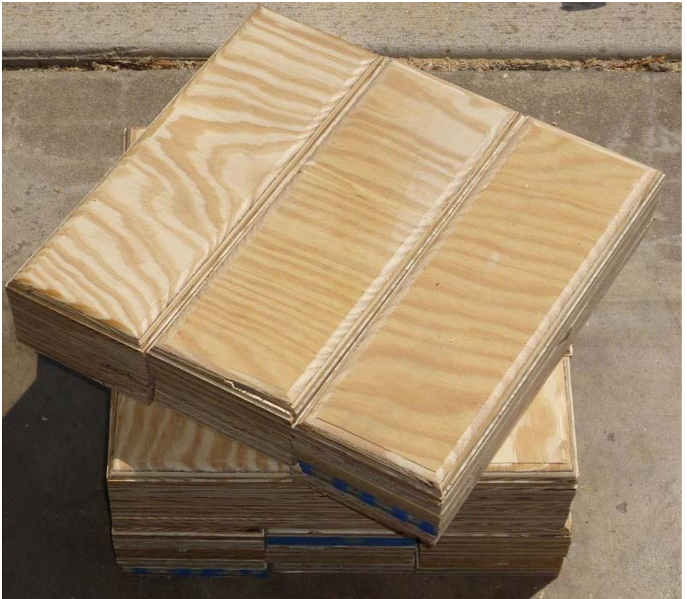
Caption: The (9) rails were glued to the 3/4" plywood floor. Each was then screwed together with (3) 3" screws.
